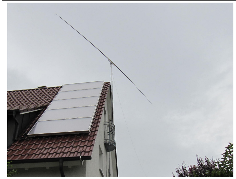
A rotary 4-band dipole above the roof
